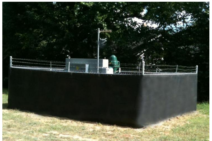
Commercial Installation around electrical Equipment
